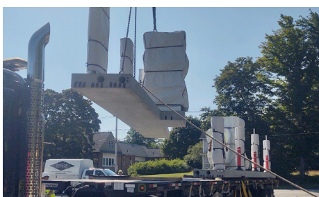
Prefabricated supercharger construction at Templeton MA
